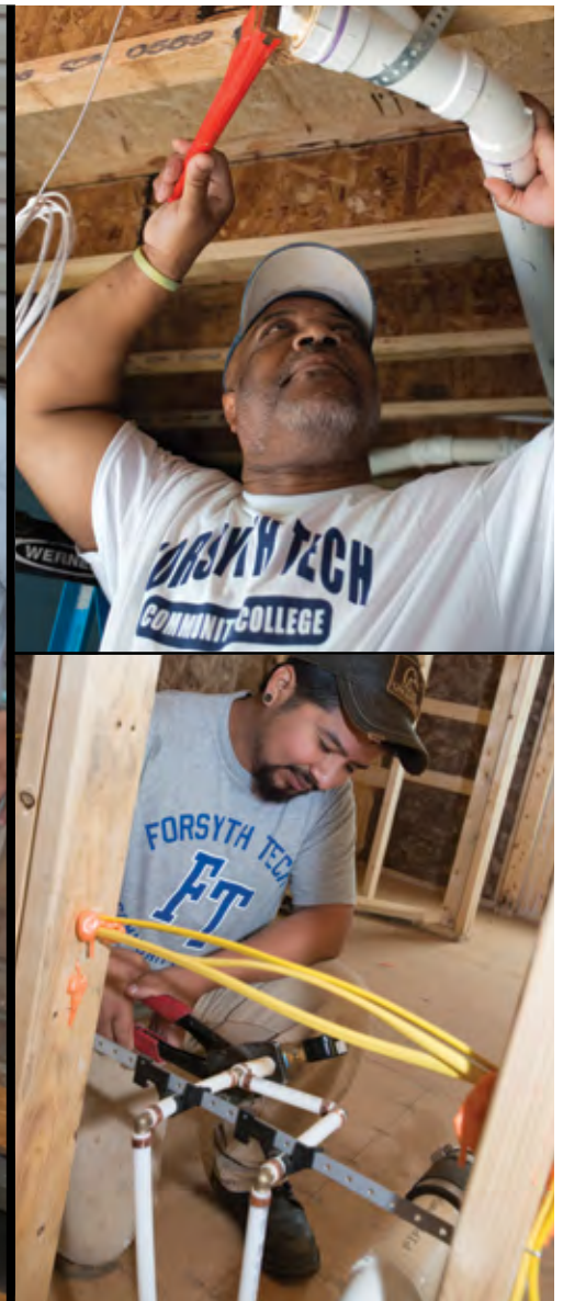
Forsyth Tech Plumbing students help build a Habitat for Humanity house.
